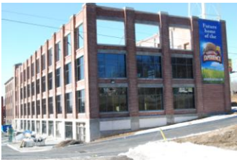
Turkey Hill Experience during renovation
