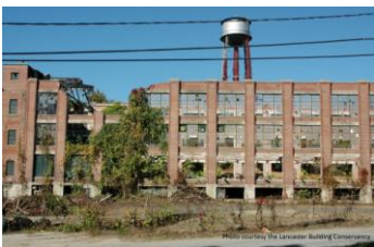
Ashley and Bailey Silk Mill prior to renovation
